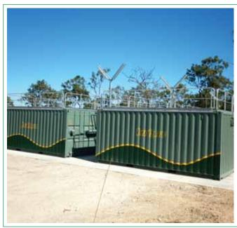
The Ozzi Kleen transportable containerised system is becoming the preferred treatment plant for mining and construction projects in remote locations – when delivered, the system can be installed and ready to operate quickly. The Ozzi Kleen transportable containerised range is available in many configurations with the modules in parallel or in series to cater for higher BOD and hydraulic loadings.
