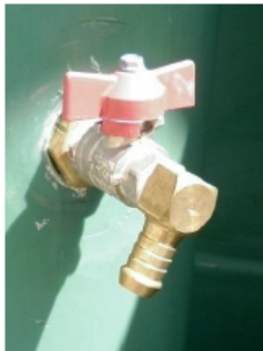
Photo 4. SK20A test tap
